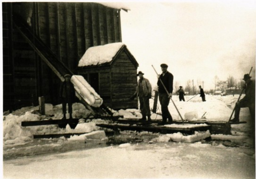
Block on the hook, pulled up to be stacked, Ephraim Jacobsen - right
